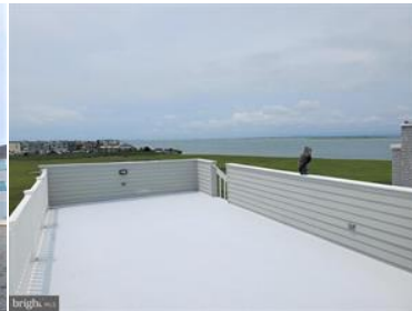
Roof Top Deck
