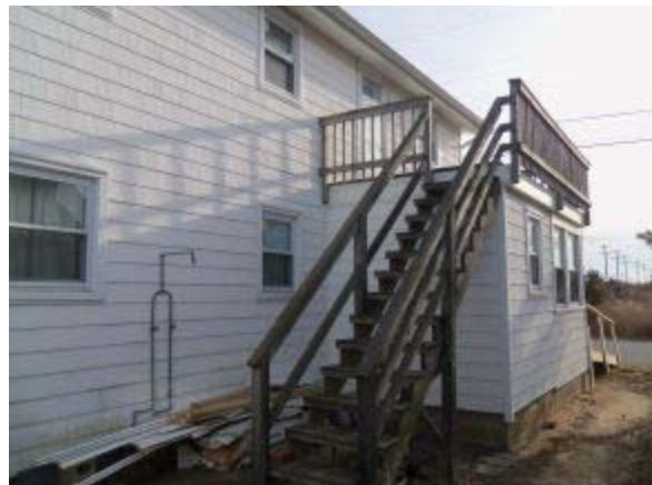
Steps to second floor deck
