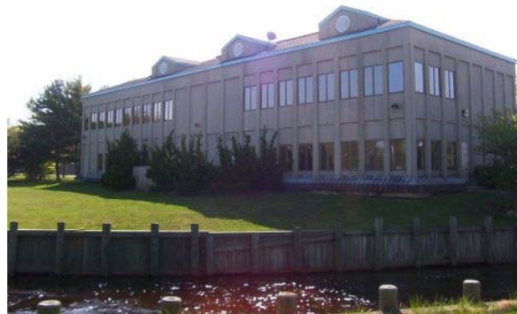
Bulkhead is not on property
