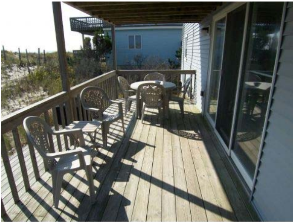
1st Floor Deck
