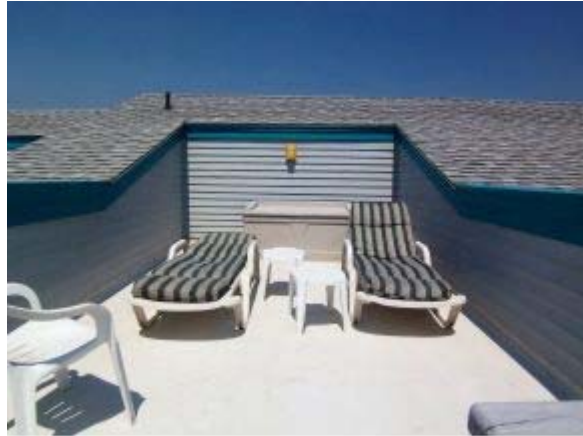
roof top deck
